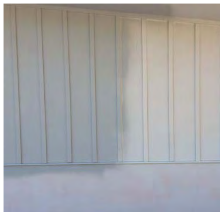
At Orinda Intermediate School, a fresh coat of Bulldog gray paint (left) contrasts with the Navajo white color formerly used on all Orinda schools.
